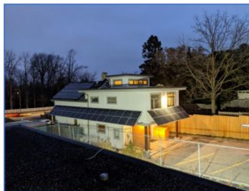
Figure 17: Residential Wall-mounted Solar PV system - courtesy of Blue Water Energy
