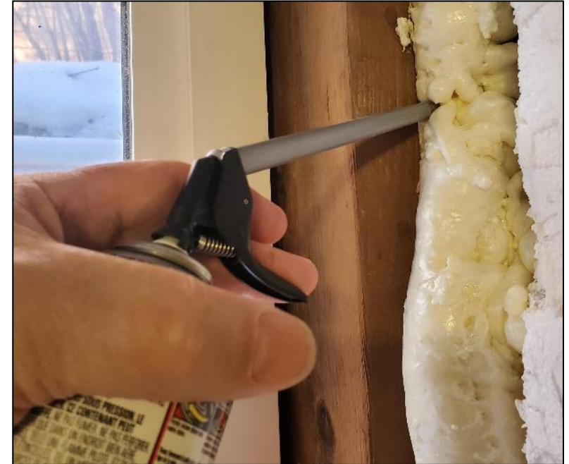
Spray foam Semi absorbent airtight
