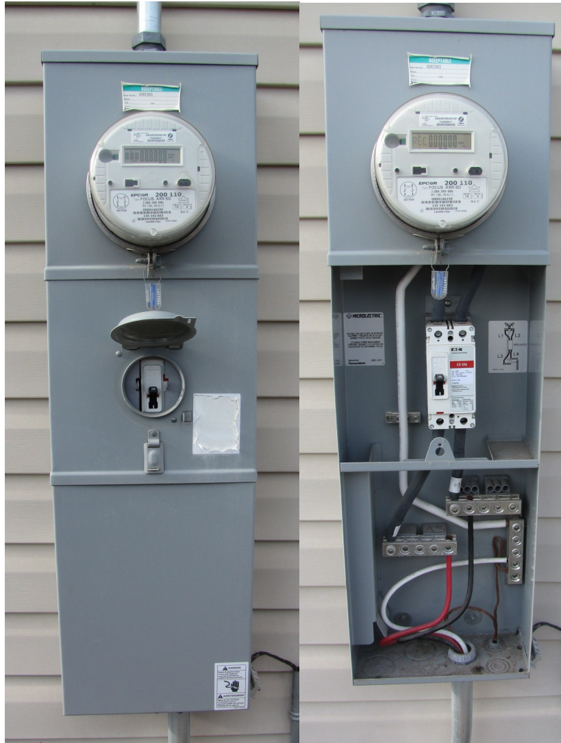
Photo: Microelectric C02M series meter sockets with splitter 200-a-120-240-v-co2-series.pdf (tnb.ca)
