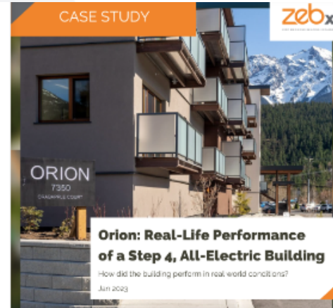
Case Study: Orion – Real-Life Performance of a Step 4, All-Electric Building
